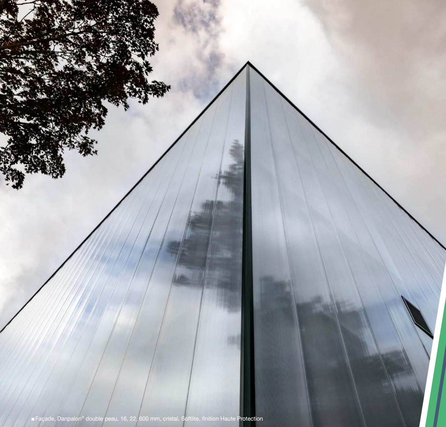
■ Façade, Danpalon® double peau, 16, 22, 600 mm, cristal, Softlite, finition Haute Protection
